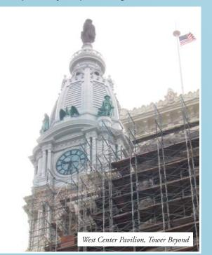
Phases 1 and 2 have been completed and work is underway on Phase 3, beginning at the Southwest Corner Pavilion. The goal of the rehabilitation is to add 50 years of serviceability with ordinary maintenance.
