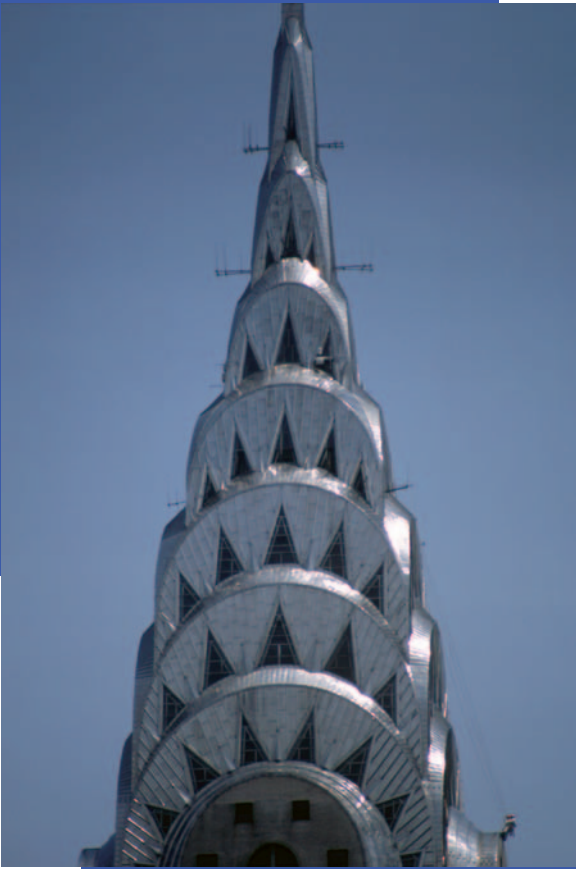
Water infiltration and existing conditions study at the Chrysler Building, New York City.
