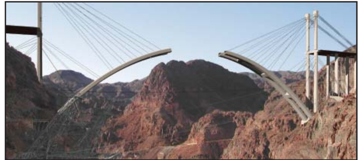
Figure 8: Alternative erection scheme
