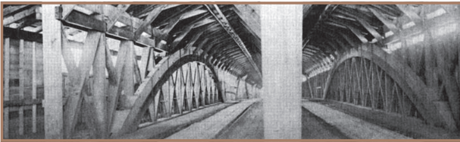
Interior of double barrel bridge showing arch and truss work.
