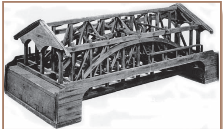
Model of Burr Truss built well into the 20th Century.
