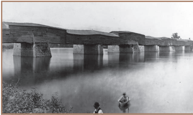
Schenectady Bridge fully covered with additional four piers
