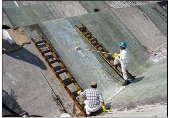
Figure 5: GFRP Bi-directional Shear Strengthening.
