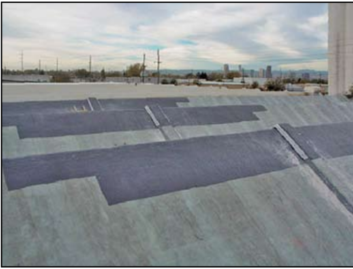
Figure 3: CFRP Negative Moment Strengthening.
