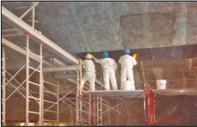
Figure 4: CFRP Positive Moment Strengthening.
