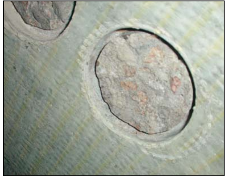
Figure 8: ASTM D4541 Testing of Bond Critical FRP.
