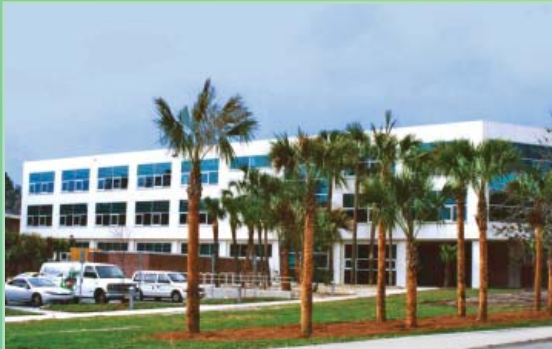
At the University of Florida's Rinker Hall — a LEED Gold Building and AIA/COTE Green Project Award Recipient — moment connections were used to provide open bays which facilitate future expansion and adaptability. Image courtesy of Walter P. Moore.
