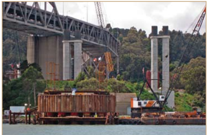
Figure 5: T1 Foundation (W2 Pier in Background).
