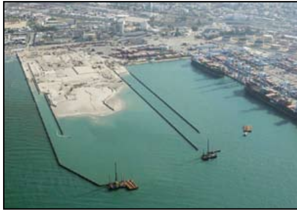
Figure 6: Overall view of sheet piling and reclamation during construction
