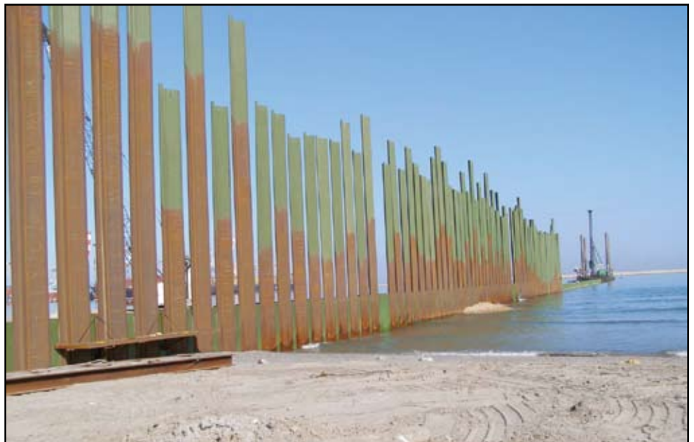
Figure 4: Sheet pile installation along retaining structure
