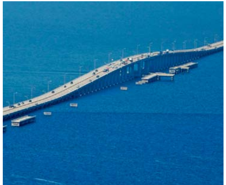
Section of Bridge Destroyed by 'Ivan'.
