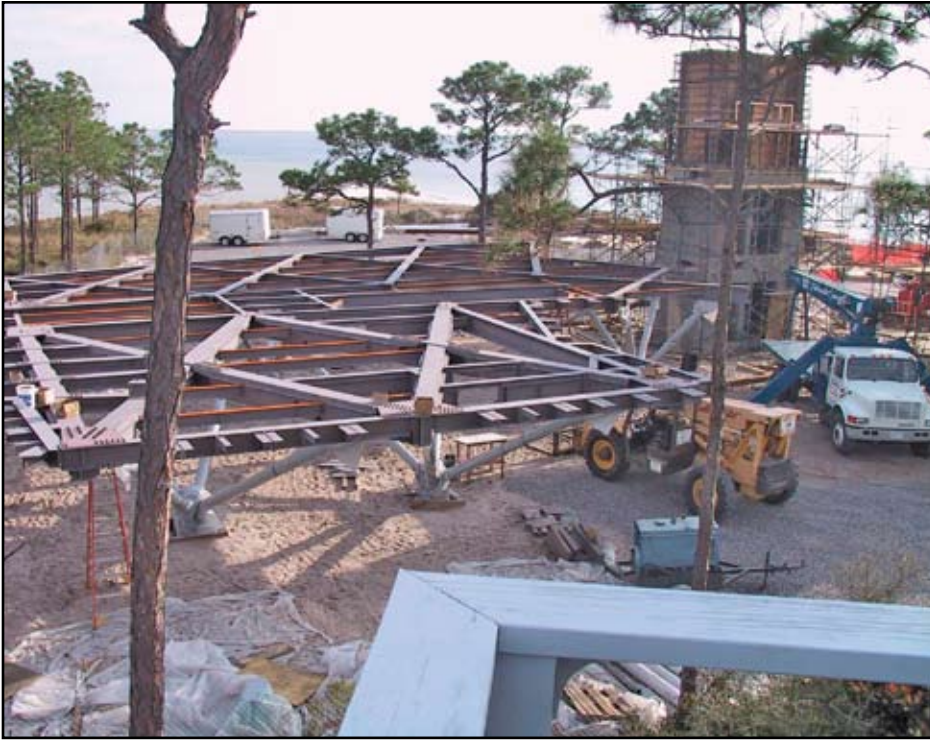
Structural Steel 1 st Floor Diaphragm Supported on Sprouts.
