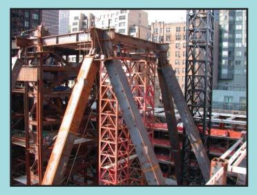
The inherent lateral stiffness and strength of the diagrid provided a significant advantage for the general stability requirement for the tower under gravity, wind and seismic loading. This resulted in a highly efficient structural system that consumed 20% less steel material in comparison to conventional moment frame structures.
