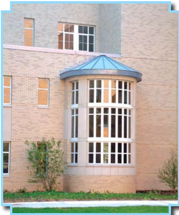
Brick veneer over CMU infill for a university building.
