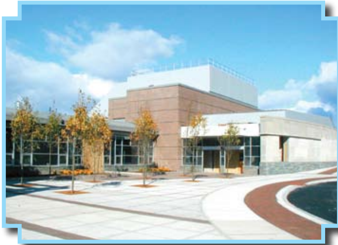
Brick veneer over CMU infill walls for a school.
