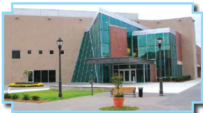
Brick veneer over CMU infill walls for a hospital.
