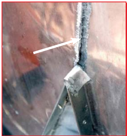
Cracked solder
