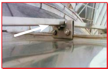
Snow stop (part of the Replaced Simple Arch Cladding)
