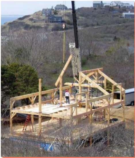
Figure 4: Cranes are used to erect frames
