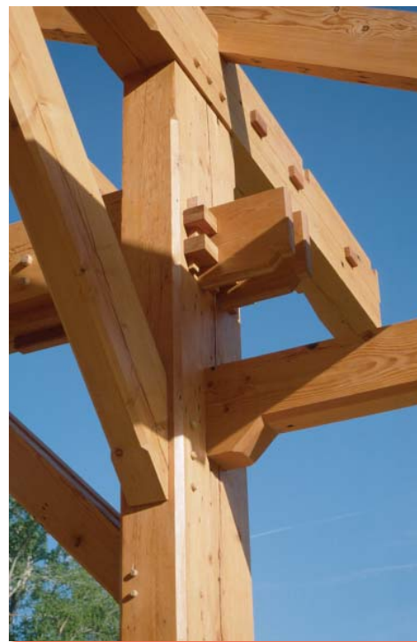
Figure 6: Modern timber joinery
