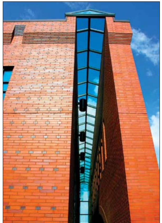
The skylight provides a covered entry while allowing natural light to fall upon the masonry detail.
