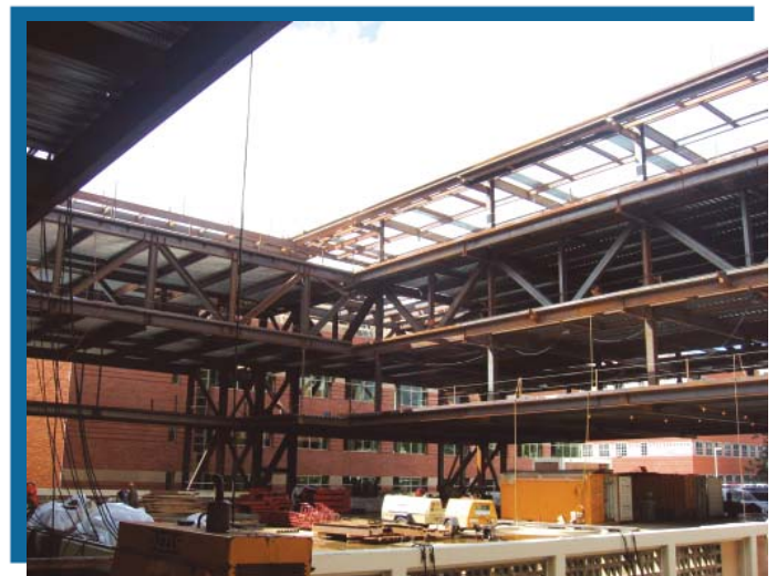
Structural view of interior courtyard
