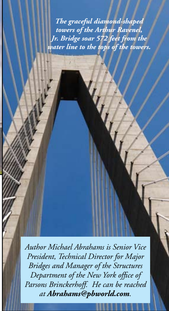
The Arthur Ravenel, Jr. Bridge over the Cooper River stretches 3.5 miles Charleston to Mount Pleasant and includes a 12-foot-wide walkway/ bikeway that provides spectacular views of the surrounding area.
