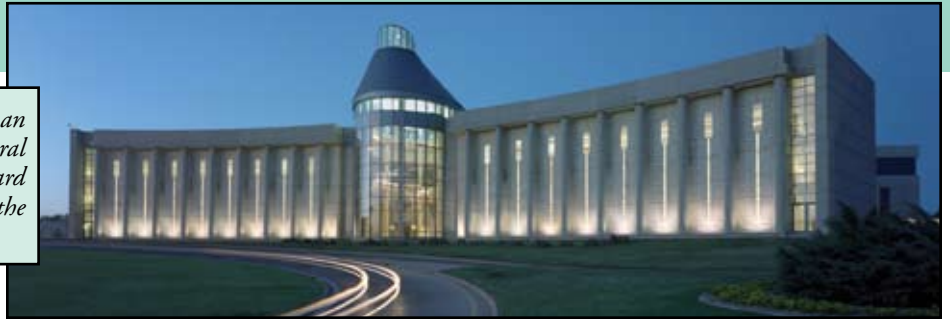
Exterior of Gallery Wings, showing Grand Hall and backlit onyx lanterns. Photo © Tim Hursley
