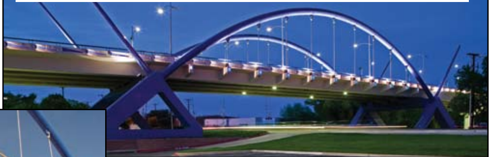
The 170-foot Arapaho Bridge is illuminated with specialty lighting. Courtesy of www.dave-lawrence.com .
