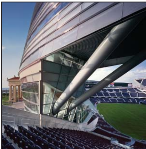
Pipe supports of the North Scoreboard. Photo courtesy ©David B. Seidel/Defined Space, Chicago.
