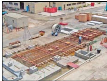
Figure 3: Replacement reinforcing bars in place
