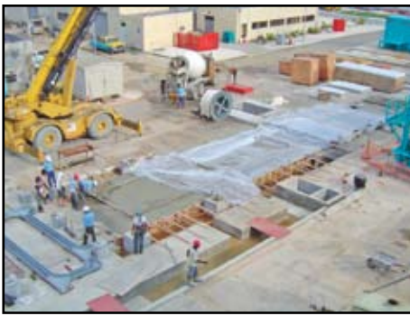
Figure 5: Final stages of repair construction
