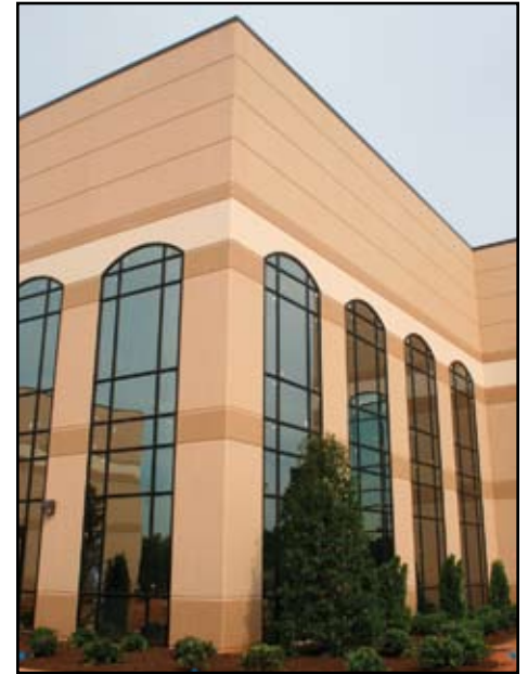
With R-values as high as R-24, this 138,400 square-foot beverage distribution center uses carbon fiber-reinforced panels to reduce the energy expended by the refrigeration system.
