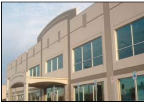
The 332,000 square foot Cardinal Health office-warehouse features carbon-fiber-reinforced wall panels up to 51 feet in height. They deliver a healthy R-16.
