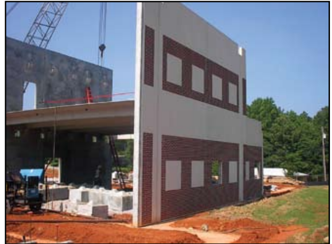
This elementary school near Greenville, S.C., incorporates thin brick on panels that use carbon fiber grid as a shear truss between the inner and outer wythes of the panel.
