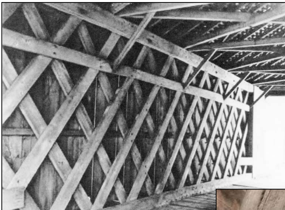
Above: Interior view of a typical "Town Lattice Truss" covered bridge. Visible are the wooden pegs used to connect the diagonal members at their intersections. Courtesy of Library of Congress-HABS/HAER.
