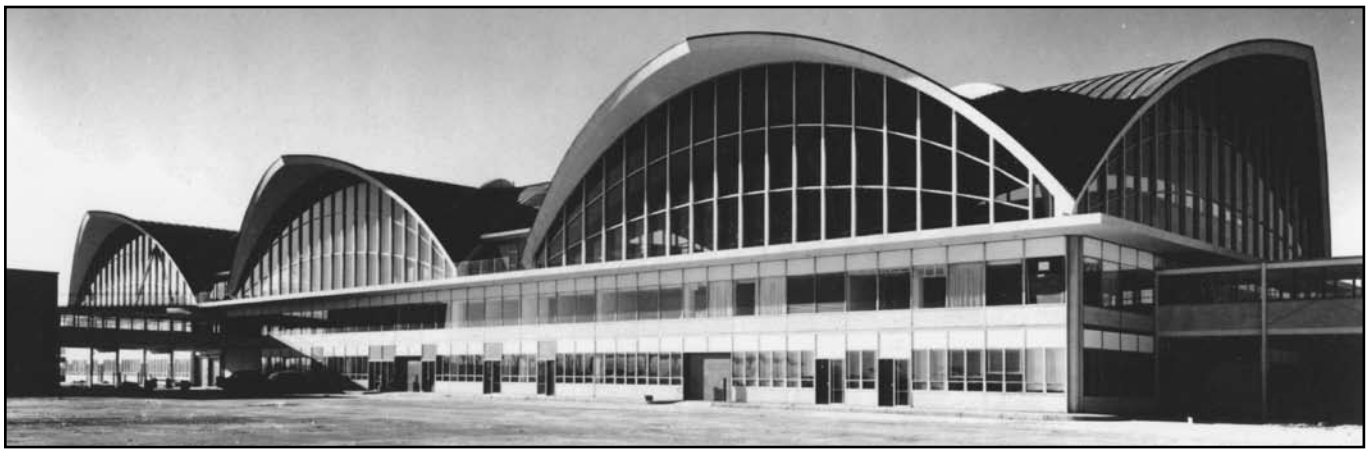
Lambert Field Terminal, St. Louis, MO (Courtesy of Princeton University Tedesko Archive)
