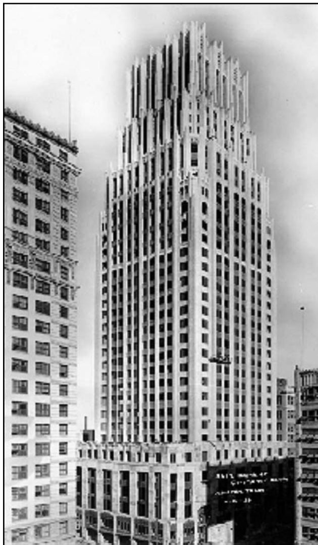
Gulf Building (JR Morgan Chase Building), Houston, Texas, 1929. The symbol of the Houston skyline for years and its tallest skyscraper from inception until 1963. Designated a National Civil Engineering Landmark in 1997. (Photo courtesy of H. Douglas Steadman)
