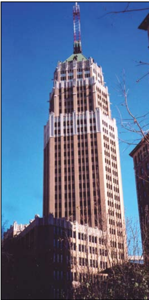
Tower Life (Smith Young) Building, San Antonio, Texas. The tallest building in San Antonio for 60 years, from 1928 until 1988. Listed on the National Register of Historic Places. (Photo courtesy of Richard Weingardt)
