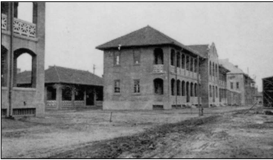
Fort Crockett in Galveston, Texas, 1909. Among the nation's very first concrete tilt-up construction projects, the first completed using design-build construction techniques. (Photo courtesy of H. Douglas Steadman)
