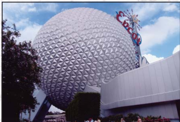
Spaceship Earth at the Epcot Center, Orlando, Florida. From opening day, Fuller's geodesic sphere served as the Center's theme structure. Photo courtesy of Richard Weingardt Consultants, Inc.
