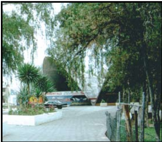
Restaurant Los Manantiales, Kochimilco, Mexico D.F., 1957-58, Architects: Joaquin and Fernando Alvarez Ordonez
