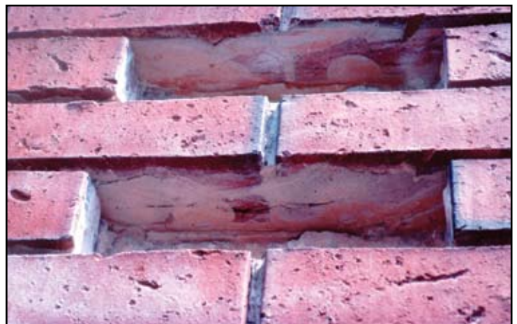
Figure 3: Brick excavation seen from the underside of the brick. Note the ragged horizontal crack through the cores of the brick
