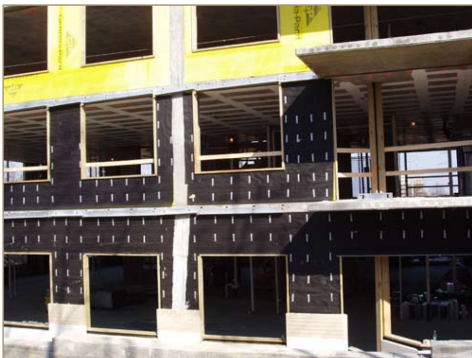
Figure 4: Steel stud backing for anchored brick veneer
