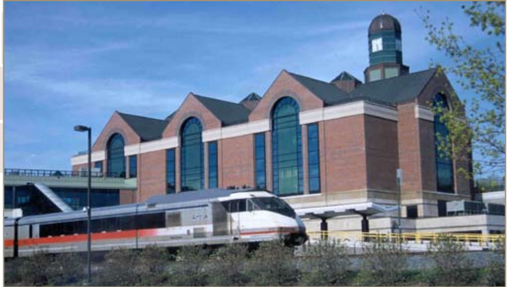
Figure 1: Train station with brick veneer (courtesy Ryan-Biggs Associates/James J. Shaughnessy)
