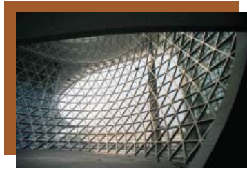
Scienceland Egg, a 164 ft wide aluminum-framed structure in Shanghai, China; photo courtesy of Temcor
