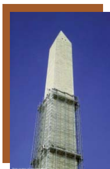
Aluminum scaffolding used during the 1997 repair of the Washington Monument
