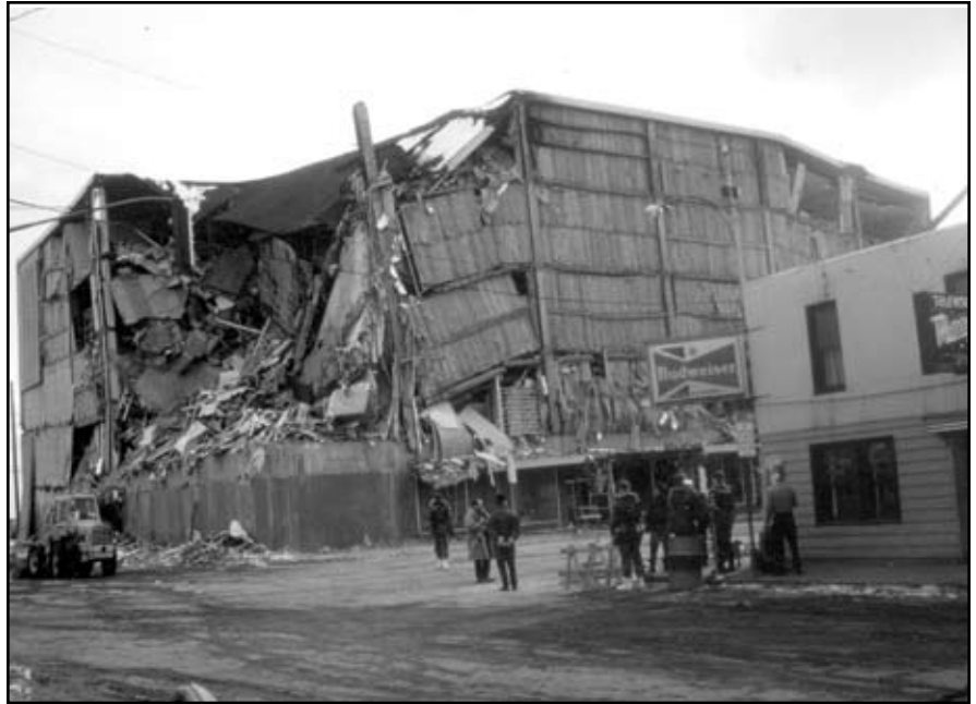
Alaska Earthquake March 27, 1964. Wreckage of the J.C. Penney Department Store at Fifth Avenue and D Street in Anchorage. The building failed after sustained seismic shaking. Most of the rubble has been cleared from the streets. Courtesy of http://libraryphoto.cr.usgs.gov .
