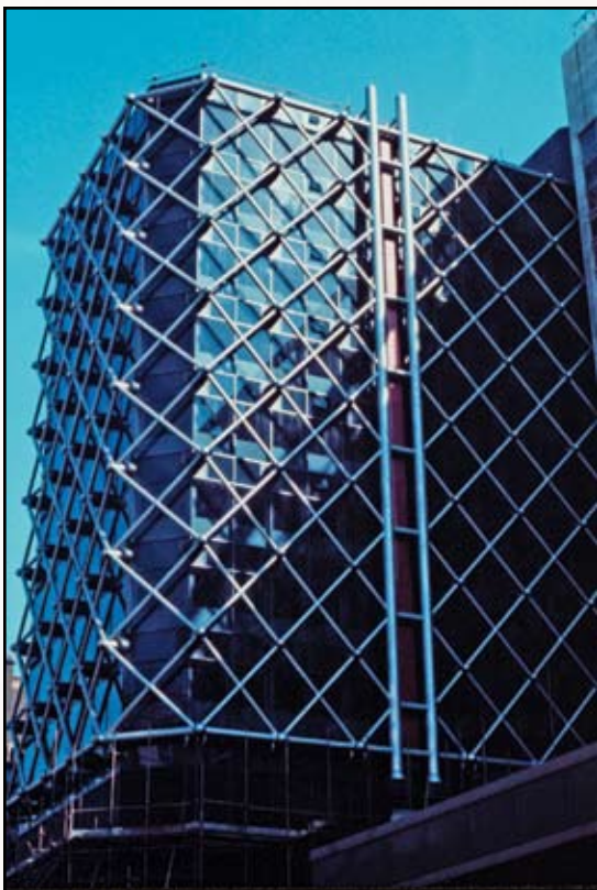
Figure 3: Bush Lane House, UK, with Water-Cooled Hollow Steel Structural Members © Arup Associates
