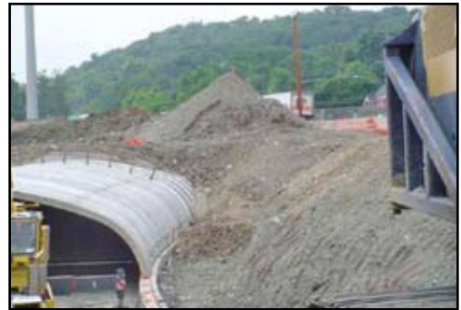
Figure 3: One of several distinct overburden stockpiles placed over the Duck Creek Culvert.
