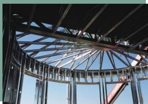
Steel framing offers the versatility of curved wall, roof, and floor systems, including the curved headers and roof trusses shown here. Specifying these systems is made easier by referencing industry approved standards.
