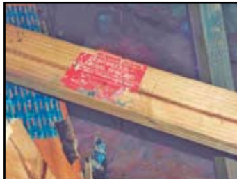
Figure 1: This building roof collapse resulted from a procedural failure in the construction and inspection of permanent bracing, despite the presence of manufacturer-installed red tags shown in the photograph on the right.
