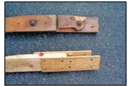
Figure 2: Comparison of original truss connection to improperly modified truss bottom chord and splice that utilized drywall screws.
