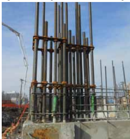
Figure 4. Example of a prefabricated shear wall cage of HPCR.
