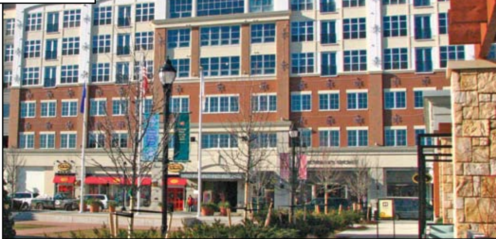
Bayshore Town Center North Parking Structure – Opening Day 2006.
