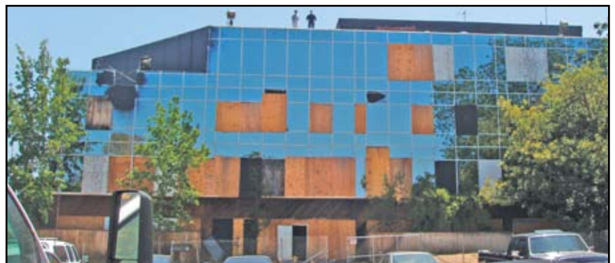
Figure 2a: West face of the Four Seasons Building
