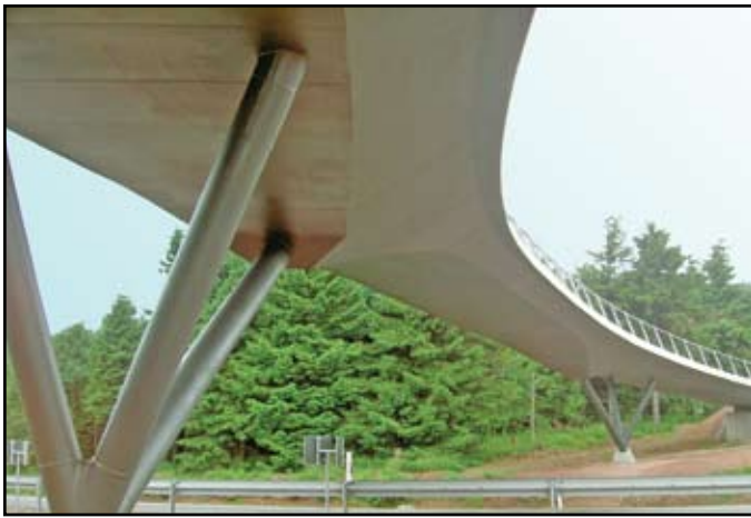
Figure 4: Rondell pedestrian variable deep orthotropic steel box girder bridge in Germany. Photo courtesy of Donges Steel Company, Germany
