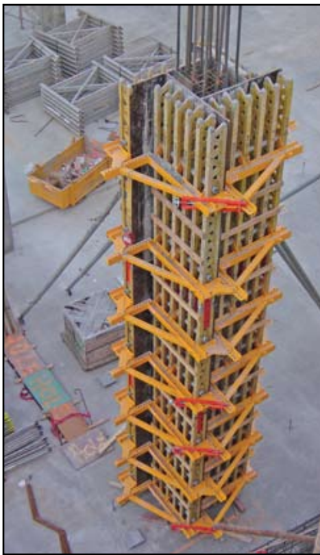
Figure 3: Adjustable column formwork
