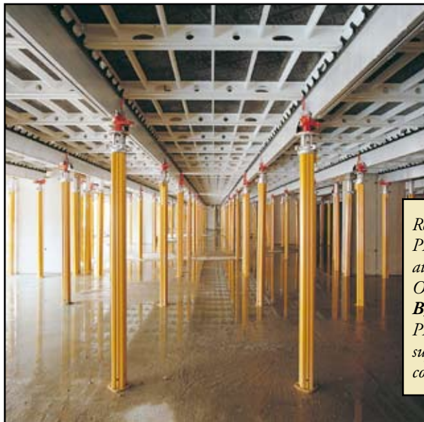
Figure 4: Light weight, quick strip floor formwork
