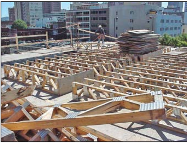
Figure 3: Beams and Girders – Same Depth.
