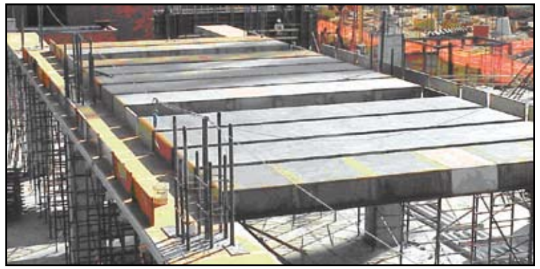
Figure 4: Large Sections of Formwork.
