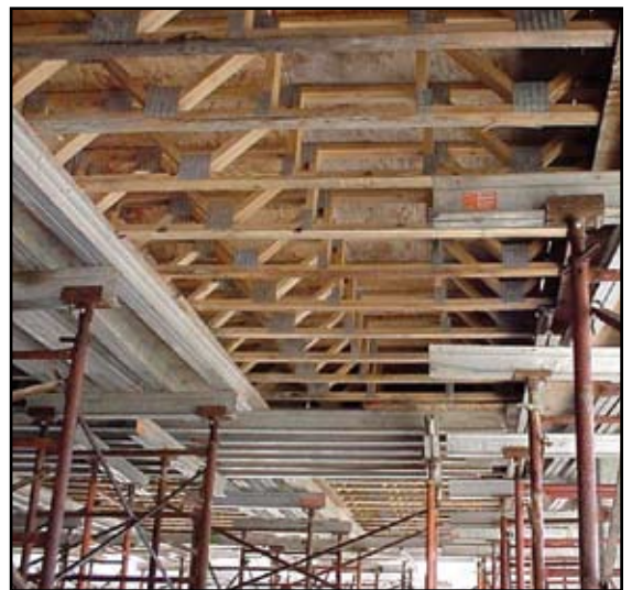
Figure 2: Formwork Trusses.
