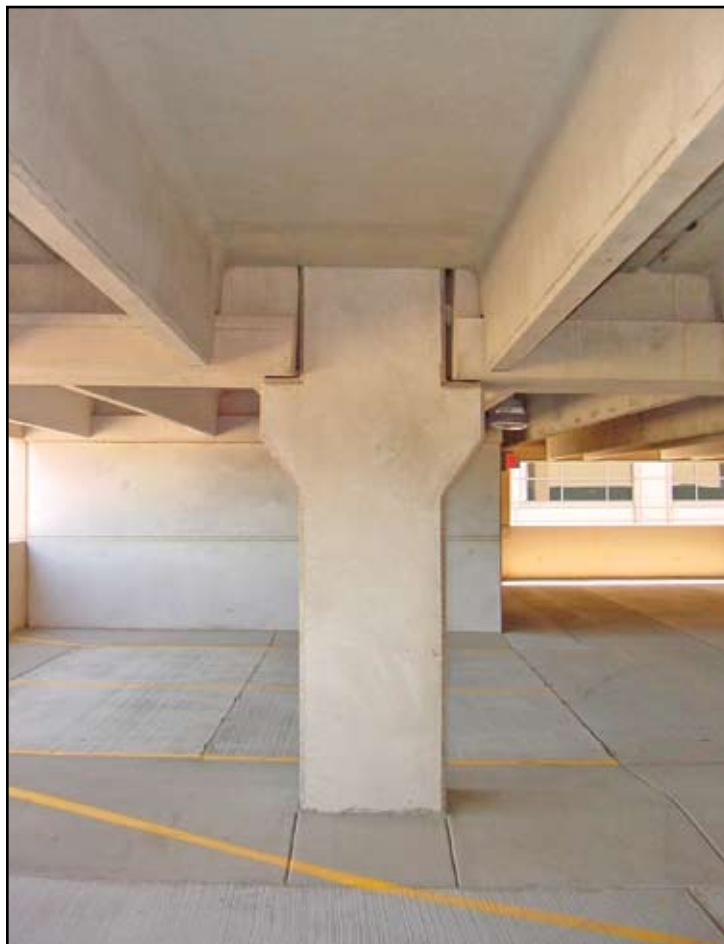
Underside of double-tee.
