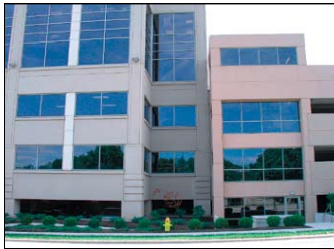
Building adjacent to parking garage.
