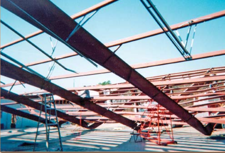
Truck garage during demolition
