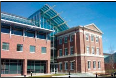
A biotechnology building whose exterior walls are brick veneer over light gauge framing.
