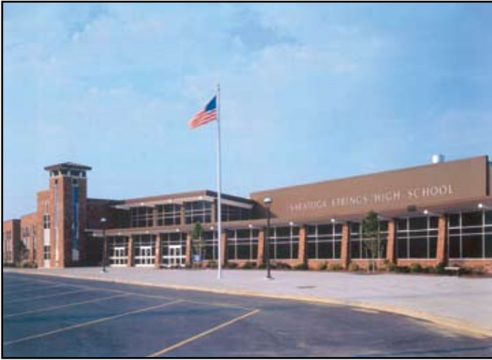
A school constructed with CMU and brick veneer walls within a steel frame.
