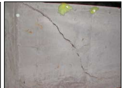
Figure 8: Significant foundation distress resulting from undesirable soil and structure interaction
