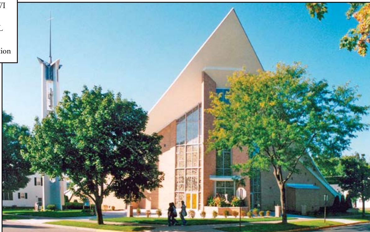
Figure 5: The Catholic Church of St. Joseph after completion of repairs.
