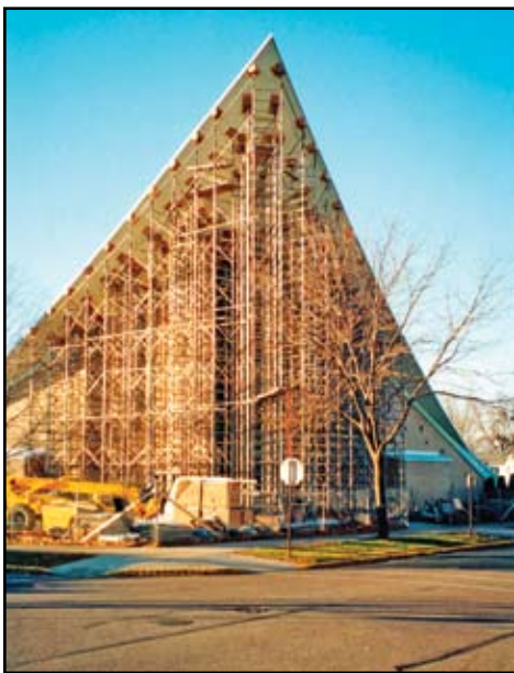
Figure 3: Shoring supporting the concrete shell roof during fin wall reconstruction.
