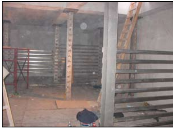
Figure 8: Damping Screen installation inside a TSD Tank. Screen geometry is designed for ease of fabrication and installation.
