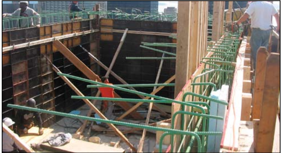
Figure 7: Constructing the TSD atop a new 60 floor residential building in New York City. The TSD tank walls were constructed with cast-in-place poured concrete, since the material and labor to install was easily obtainable.
