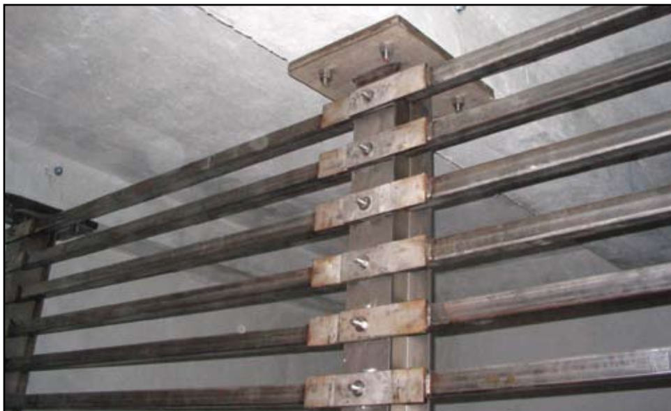
Figure 9: TSD Damping Screens are fastened to the tank roof, avoiding piercing of the waterproofing membrane.
