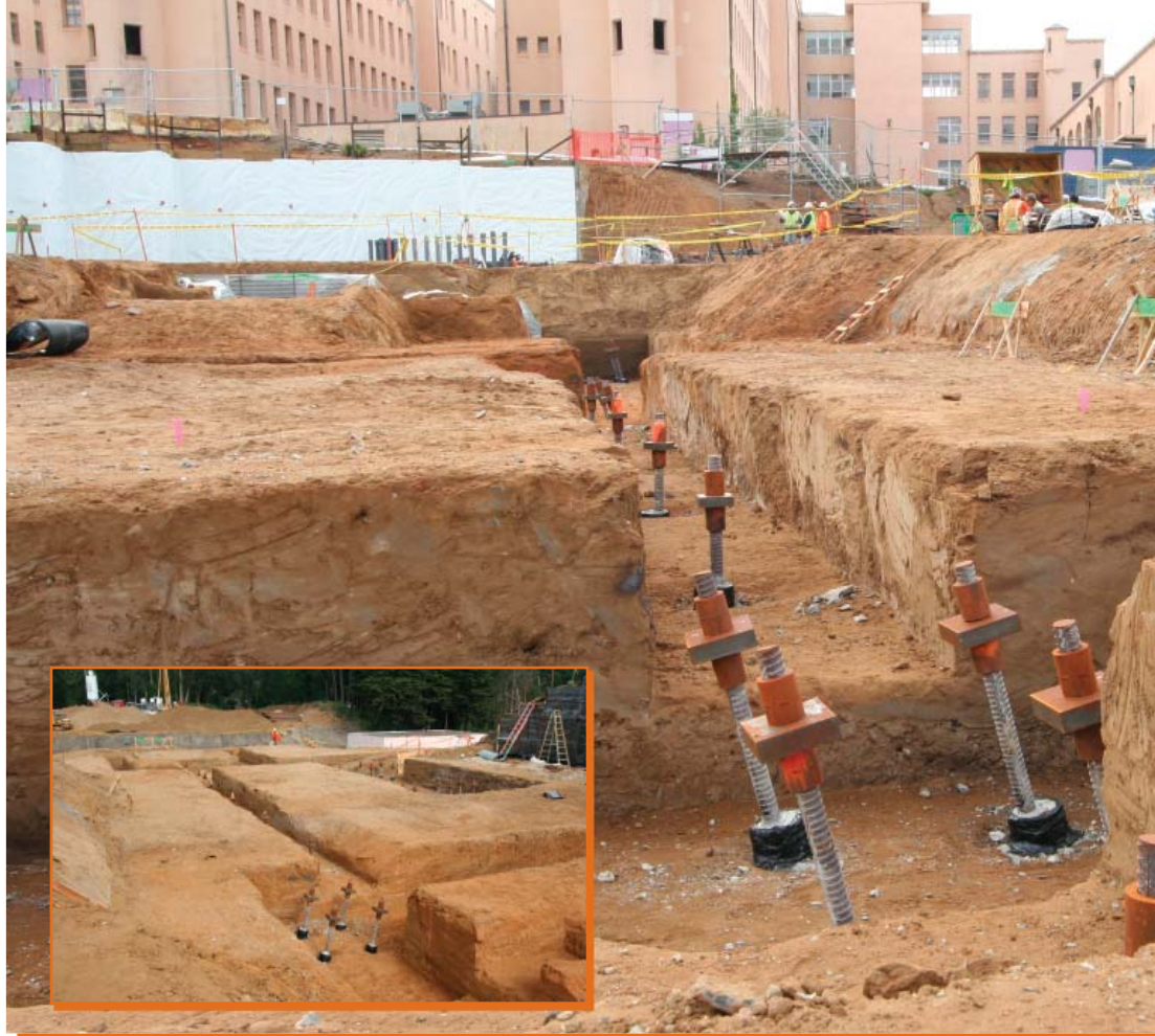
Foundation during construction (Photo Courtesy of Michelle Gale)
