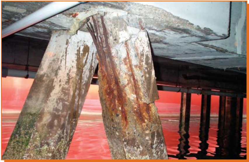
Figure 1: Too Frequently Occurring Raked Pile Configuration
