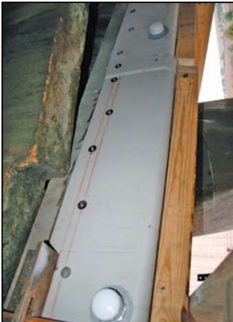
Using an aerial lift (above), the jackets were attached to the lintel beam and 4,000 psi cementitious grout was pumped through ports on the back face of the jackets (left).
