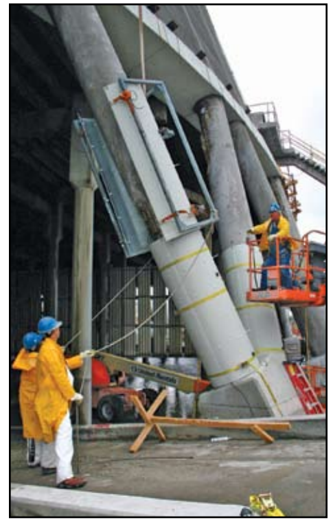
For each column, the jacket was divided into six pieces – two pieces each for the bottom, middle and top.
