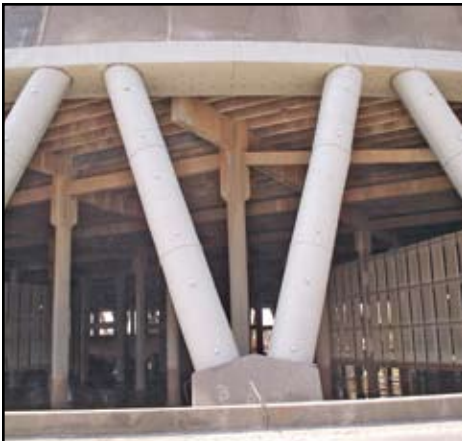
View of installed lintel beam and column jackets.
