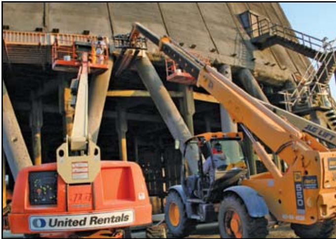
Using an aerial lift (above), the jackets were attached to the lintel beam and 4,000 psi cementitious grout was pumped through ports on the back face of the jackets (left).
