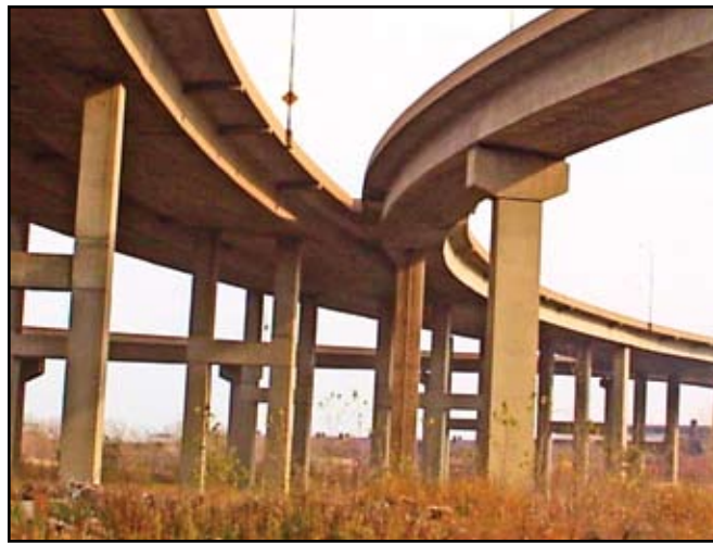
Figure 1: Cline Avenue Bridge Structures
