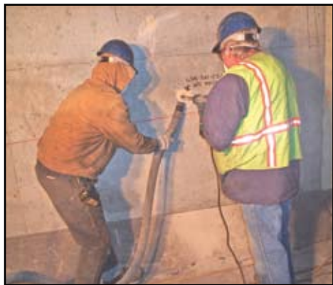
Figure 5: Crew drilling inspection hole into tendon duct
