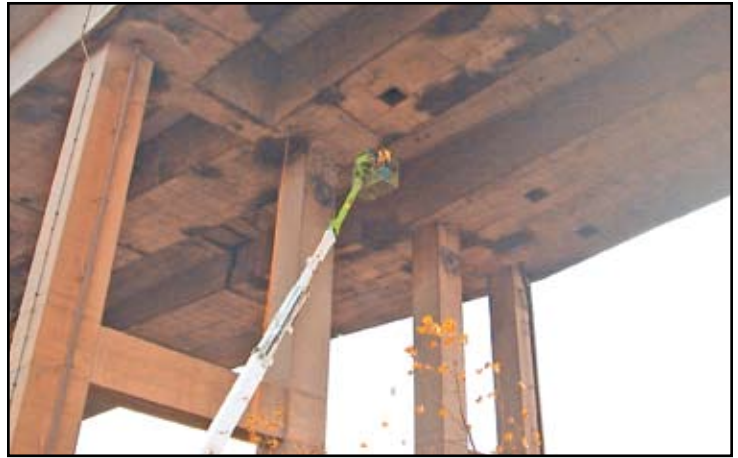
Figure 7: Access to the bridge was by 120-foot boom-lift
