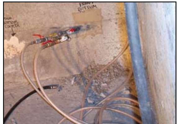
Figure 2 Hooking up vacuum grouting equipment to a tendon void
