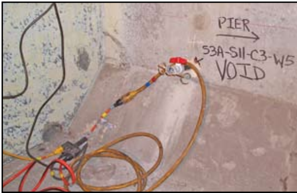
Figure 6: Hooking up vacuum grouting equipment to a tendon void
