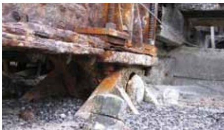
Figure 4. Hinge pin arrangement connecting the transfer bridge to the abutment.
