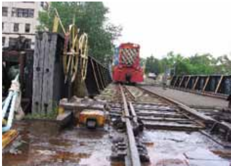
Figure 3. Toggle bars connecting the car float to the transfer bridge.
